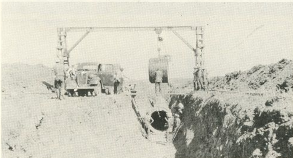
"Our CCC boys at work on the big syphon we built to connect two irrigation canals in the Bell Fourth irrigation system, near Bell Fourth, South Dakota. This concrete syphon replaced an ancient one of wood. I'm in the picture — someplace." --Albert B. Hopkins
